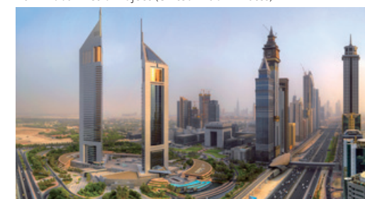
2011 Dubai Metro Project (United Arab Emirates)
