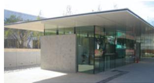
Building with exposed concrete walls made using high-quality recycled aggregate
