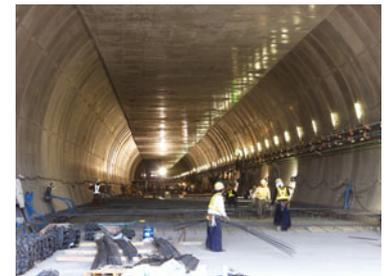
The tunnel entrance is completed after the shield machine passed through.
