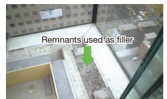
Remnants of fire-resistant covering material, effectively recycled as filler on each floor
