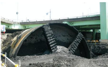
Shield machine finally arriving at ground level
