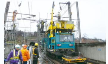
Using a road rail crane to replace overhead wire poles, in order to reopen the Tohoku Shinkansen as soon as possible.
