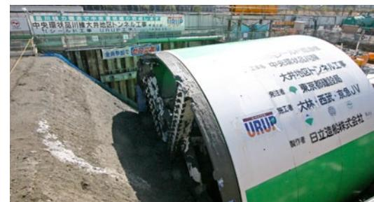
The URUP method uses a shield machine to tunnel underground through the entire length of the tunnel from entrance to exit. It eliminates the need to excavate vertical shafts.
