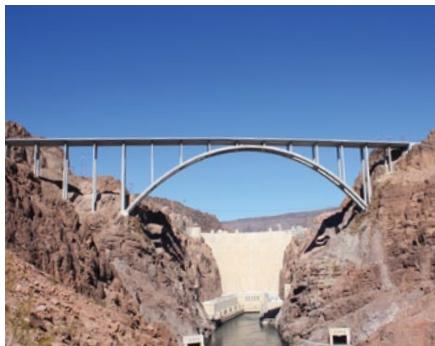
The Colorado River Bridge was constructed as a bypass for the Hoover Dam, a U.S. National Historic Landmark. A large curved arch supports the roadway deck, and construction proceeded from both ends towards the center. The bridge is 323 meters long and spans a gorge 274 meters high. This is the longest concrete arch bridge in North America and the fourth longest in the world (at the time of construction).
