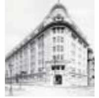
Osaka Shosen Kobe Branch building
