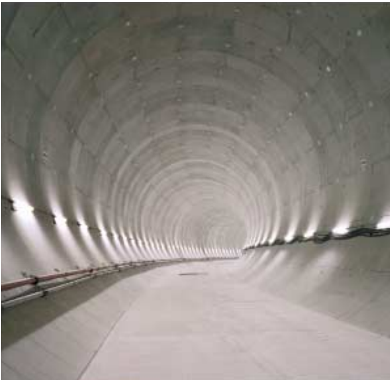
The Metropolitan Area Outer Discharge Channel - Tunnel Contract No.1
