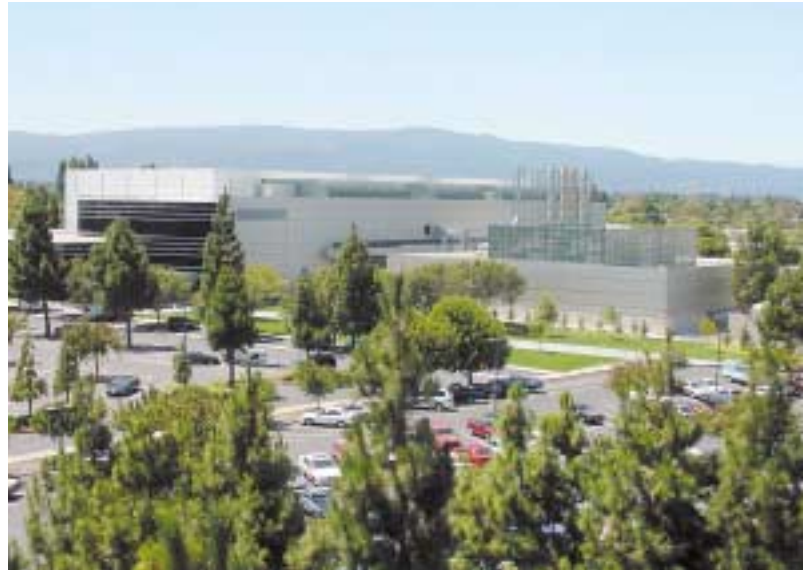
The Applied Materials technology center
