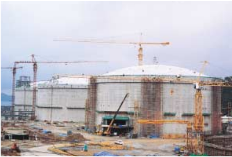
Left: Tongyong LNG Terminal (#1, 2 & 3) [South Korea] Right: Taiwan North-South High Speed Rail Project [Taiwan]
