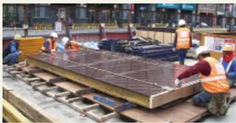
Concrete-forming panels made of 18mm-thick plywood
