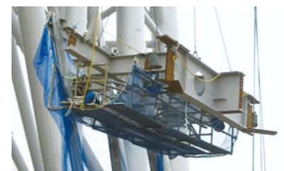
Safety nets on the steel frame are attached on the ground before being hoisted up.
