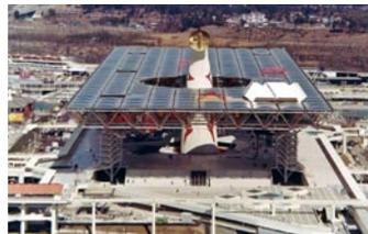
Expo '70, held under the theme of "Progress and Harmony for Mankind," was the first World's Fair held in Asia. The roof over the theme pavilion, connected with cast-iron pipes which were 290.8 meters long, 108 meters wide, and weighed 4,204 tons, was assembled on the ground, after which the whole roof was lifted up. This was the first attempt in the world of lifting up such a large structure, and attracted attention from many quarters.
