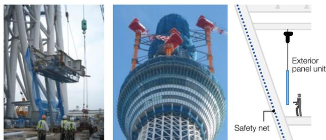
(left) Safety nets are attached to building materials at ground level. (middle, right) Once the building materials are in place at heights, work can be conducted safely within the confines of the net. In addition to protecting against falling objects, this also enables workers to carry out their job safely at unprecedented heights.
