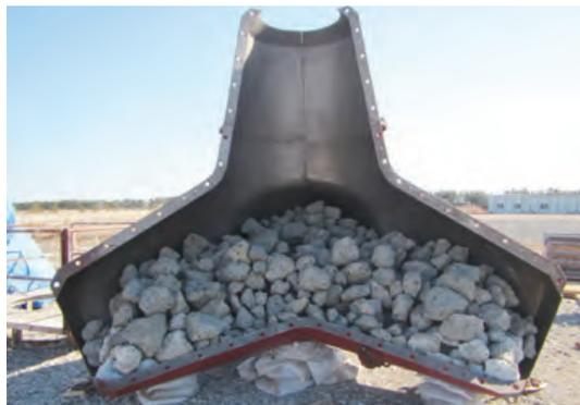
Filling a tetrapod form with concrete rubble
