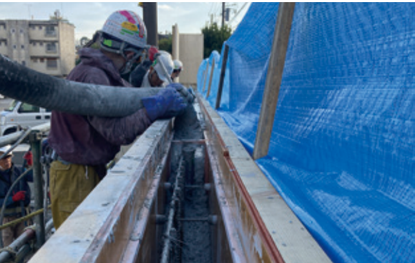
Casting concrete using a concrete pump
