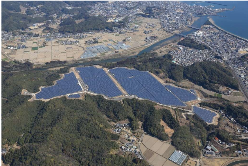
Project 03 Hyugahichiya Solar Power Station, Solar PV
