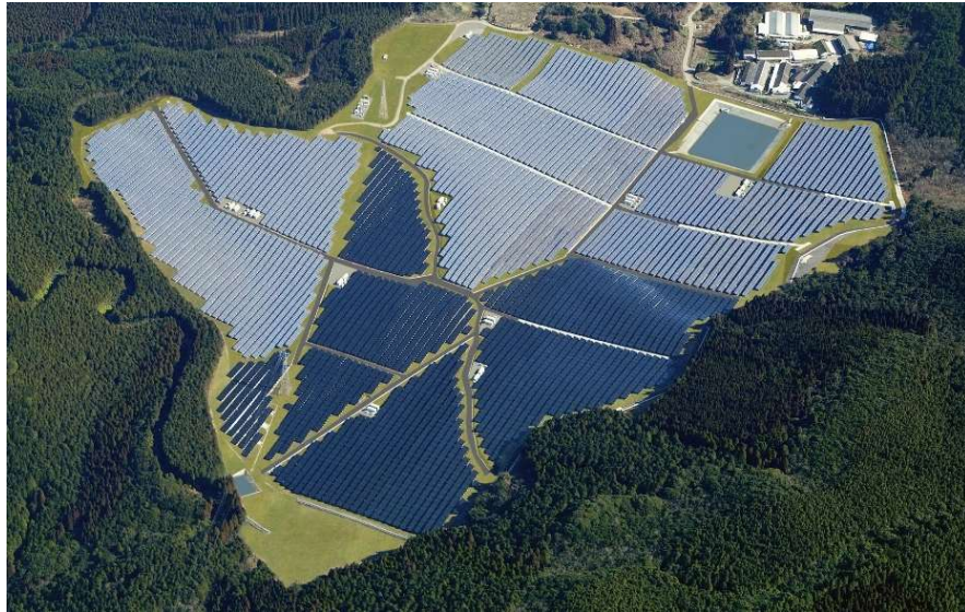
Project 01 Ashikita Solar Power Station, Solar PV
