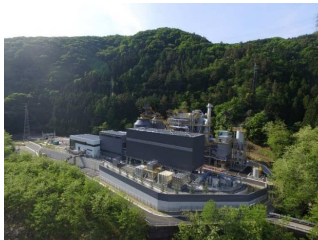
[Project 03-2 Otsuki Biomass Power Plant]
