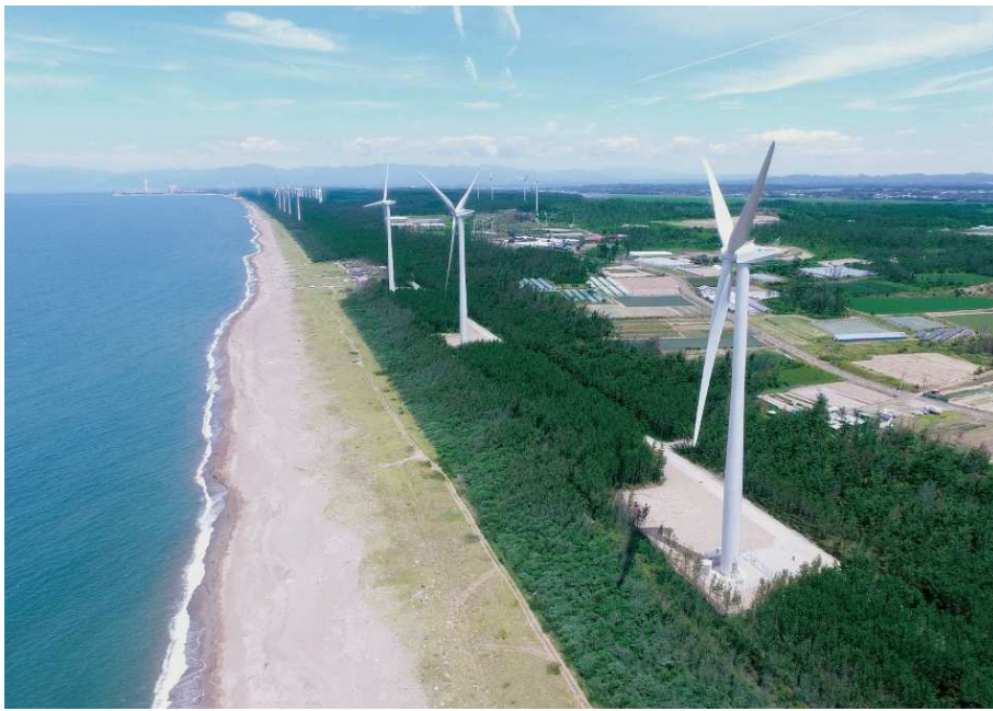
Project 04 Mitanehamada Wind Power Station
