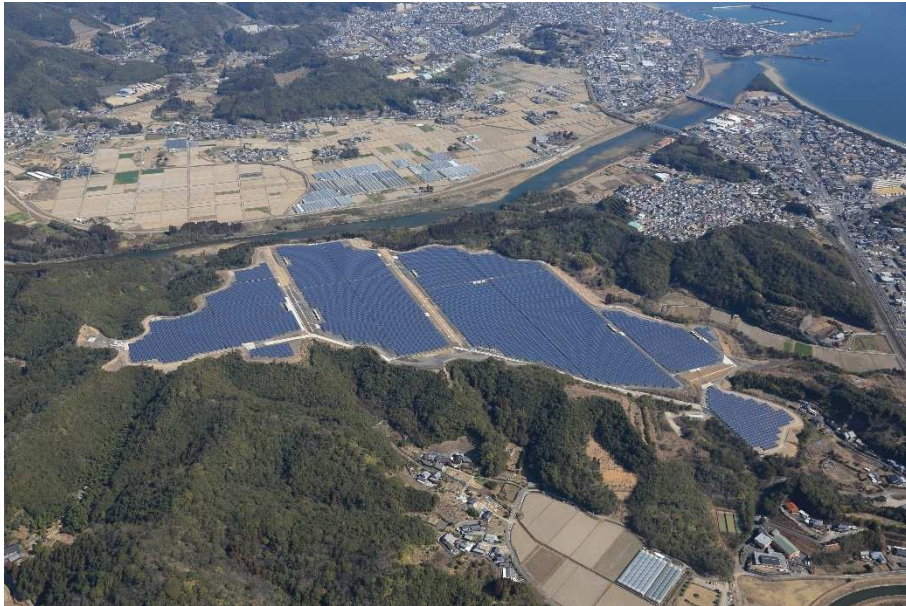
Project 03 Hyugahichiya Solar Power Station, Solar PV
