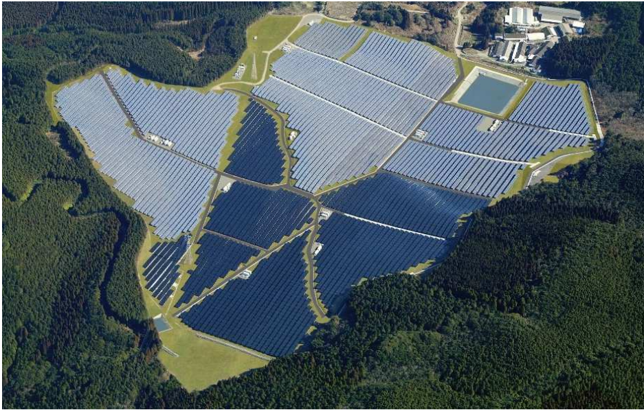
Project 01 Ashikita Solar Power Station, Solar PV
