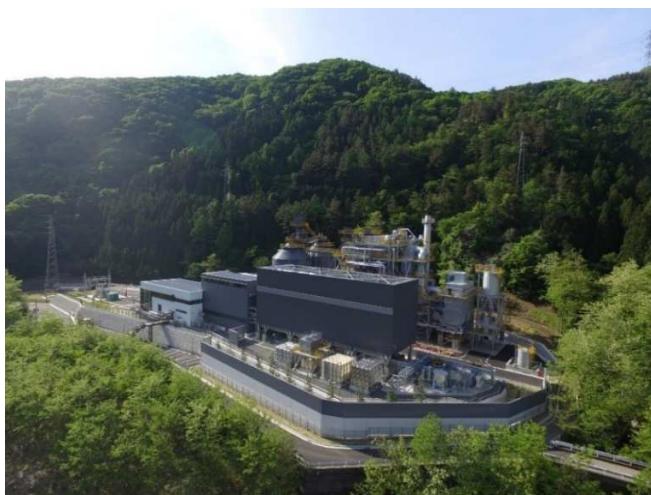
[Project 03-2 Otsuki Biomass Power Plant]
