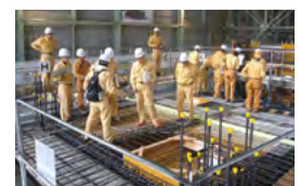
Finding multiple defects concealed in a model construction site
