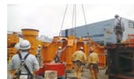
Assembling a tower crane platform
