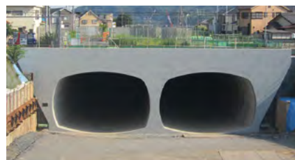
View of the tunnel entrance of the Kawajiri Tunnel at Sagami Longitudinal Expressway Project
