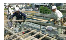
Assembling a scaffold
