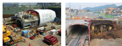
A shield tunneling machine beginning the tunnel above ground (left) and arriving at the other end of the tunnel (right)
