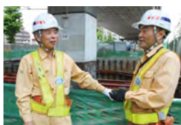
A senior employee with highly developed expertise provides on-site support as a deputy project manager
