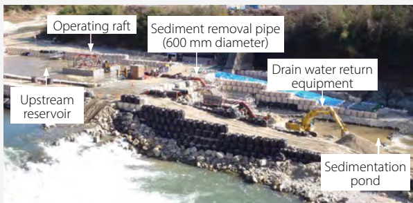
A demonstration test of using large-diameter (600 mm) sediment removal pipe to remove sediment that has accumulated at the bottom of a river
