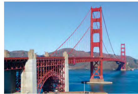
Golden Gate Bridge Seismic Retrofit (U.S.)
