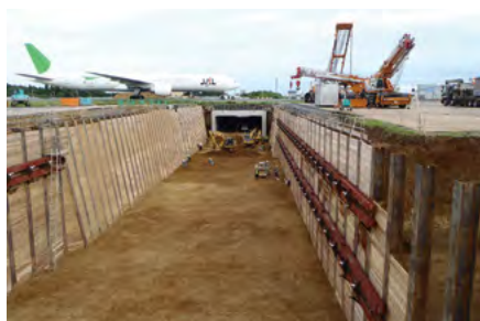
Inclined-braceless excavation support (Narita Kinone Tunnel No. 2 installation project, Narita International Airport)
