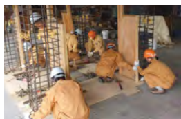
Assembling pillar reinforcement bars and concrete molds
