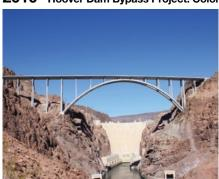
The Colorado River Bridge was constructed as a bypass for the Hoover Dam a U.S. National Historic Landmark. A large curved arch supports the roadway deck, and construction proceeded from both ends towards the center. The bridge is 323 meters long and spans a gorge 274 meters high. This is the longest concrete arch bridge in North America and the fourth longest in the world (at the time of construction).
