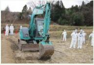
Decontamination work removing topsoil using heavy equipment
