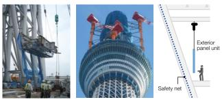
(left) Safety nets are attached to building materials at ground level.
