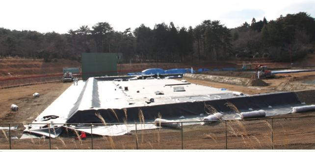
Temporary storage site constructed on a municipal baseball field in Okuma, an important facility for storing debris and items to be disposed of as a result of the decontamination work
