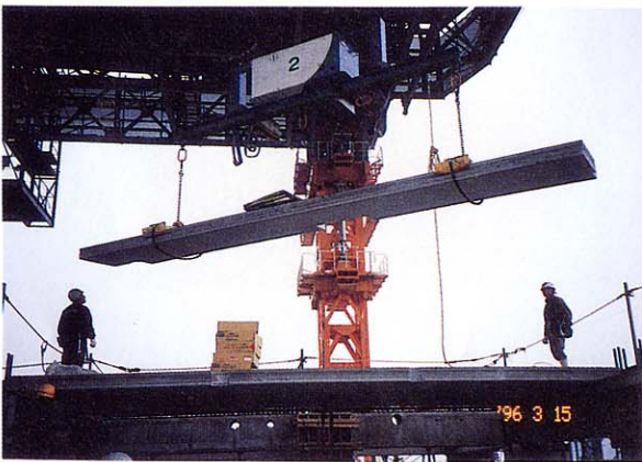
Photo 2 床版の敷設状況 Installation of Slab PCa
