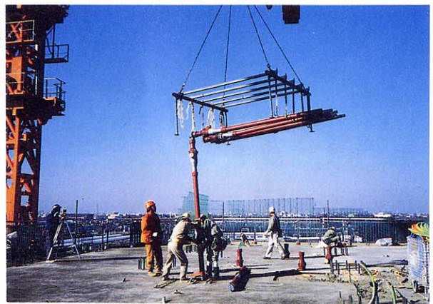
Photo 3 排水縦管の取付け Setting of Vertical Sewer Pipes
