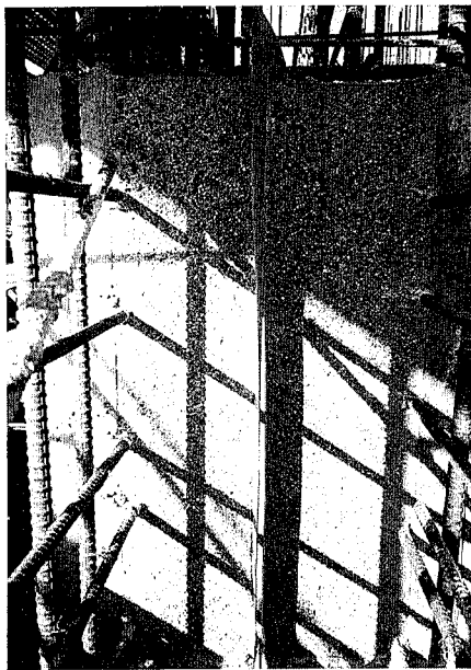
Photo 5 洗出し完了 Concrete Surface of Green Cut (Ex.2)
