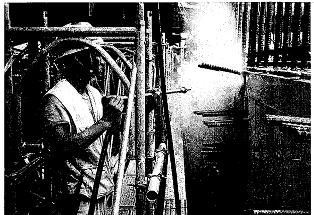
Photo 3 洗出し状況 Green Cutting Work
