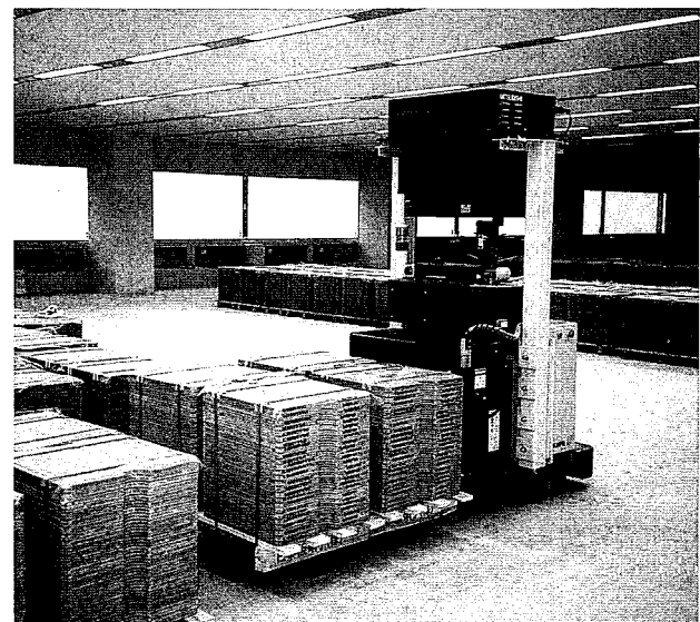
Photo 4 OAフロアの搬送 OA Floor Transportation
