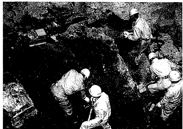
Photo 1 現位置調査状況 In-site Tests View in the Vertical Shaft
