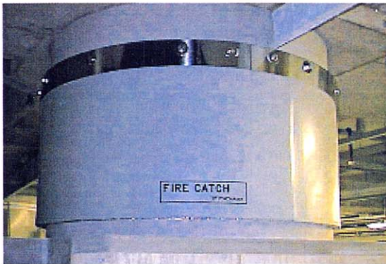
Photo 4 耐火被覆外観 Appearance of Fire Protection System "Fire Catch™"
