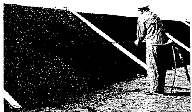
Photo 1 緑化基盤材の吹付け状況 State of Spraying Plants Growth Base
