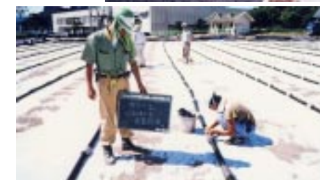
Photo 7 GOALパイプ敷設 GOAL Pipe Setting
