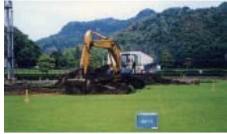
Photo 1 鋤取り撤去 Surface Cutting
