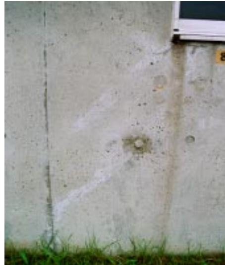
Photo. 7 ひび割れ補修後の状況 Appearance of Crack Repaired
