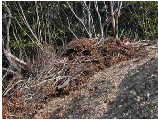
Photo 1 伐採材垣根工法とウッドチップマルチ工法 Felling Material Fence and Wood Tip Mulch
