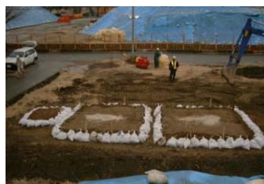
Photo 3 埋戻し（盛土）の状況 Appearance of Reclamation in the Field
