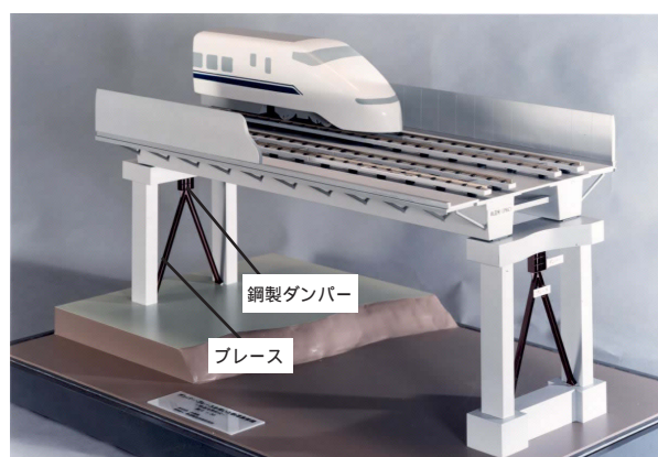
Photo 1 構造概要 Outline of The Structure
