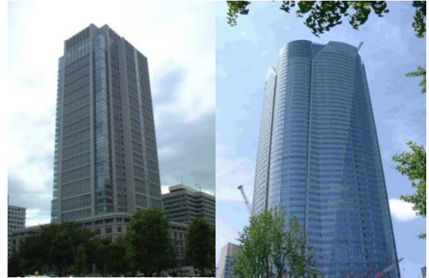
Photo 1 施工例 Example of Construction
