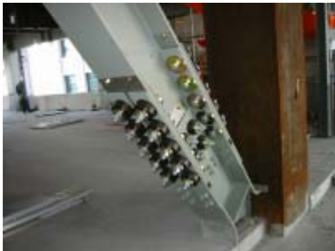
Photo 5 適用状況 Application to the Building
