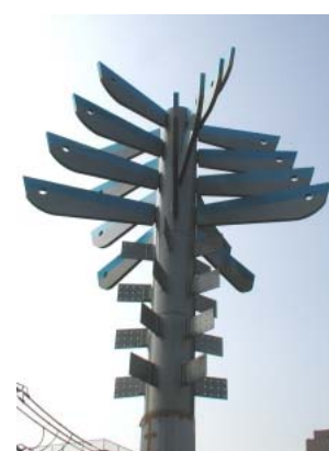
Photo 4 PLAZA FISH 現場組み立て作業中 Assembly Work Inside at Site
