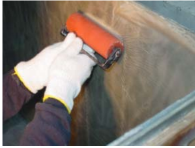
Photo 5 脱泡 Removing Entrapped Airs under Prepreg
