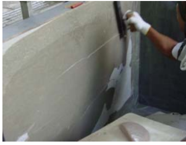
Photo 3 パテの塗付け Putting Putty on a Substrate
