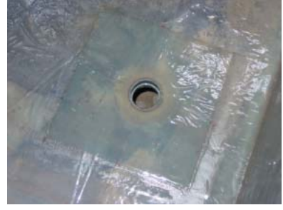
Photo 7 ドレン回り Waterproofing around a Drain
