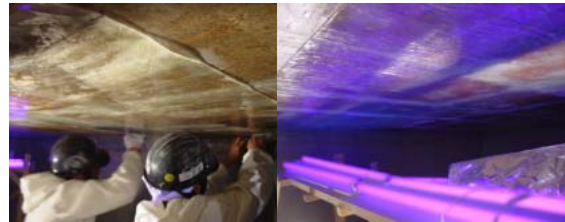
Photo 8 現場施工の状況 Execution of Qu 2 System in the Field
