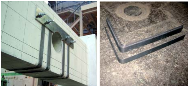
Photo 3 補強状況 View of Strengthening Portion Photo 4 L型CFRP板 L-Shaped CFRP Plate
