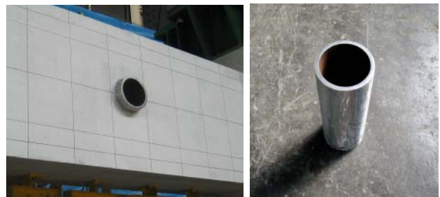
Photo 5 補強状況 View of Strengthening Portion Photo 6 鋼管 Steel Pipe
