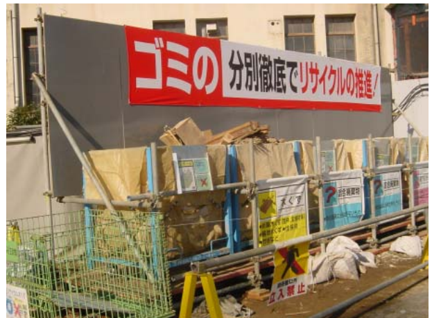
Photo 2 廃棄物置き場の状況 (大規模現場) Construction Waste Yard (Large Construction Site)
