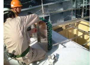
Photo 4 周期調整蓋取付 Setting of Adjuster Board
