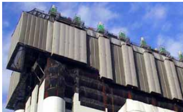
Photo 1 外周架構 Surrounding Walls
