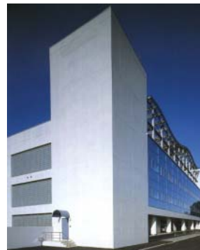
Photo 1 建物外観 Building Externals
