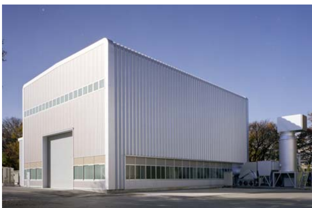
Photo 1 火災工学実験棟の外観 External Appearance of Laboratory
