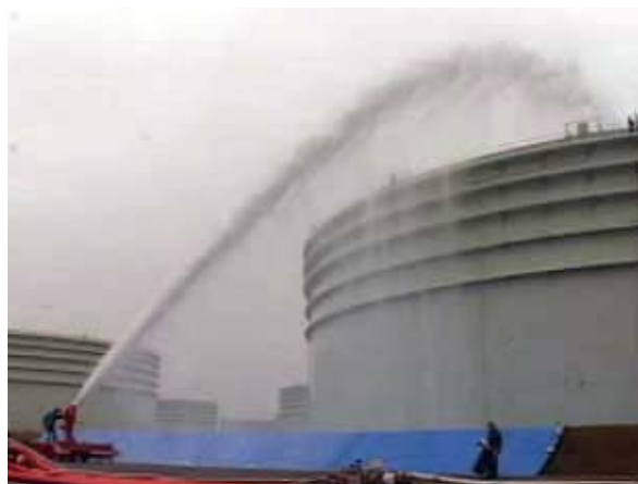
Photo 4 大容量泡放射システムの放射状況 The Largest Fire Extinguishing System for Oil Tanks by Large Quantity of Chemical Foam
