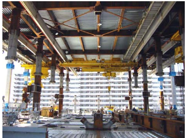
Photo 2 SCF下部の施工環境 Construction Environment below the SCF
