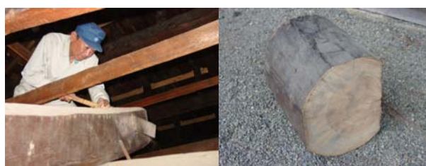
Photo 7 小屋裏での部材採取 Cutting a Part of Wood Member in Attic Space
