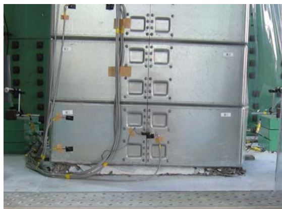
Photo 5 8 y時の塑性ヒンジ部状況 (LD試験体) Circumstances of Prastic Hinge at 8 y(Specimen LD)
