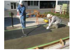
Photo 1 施工状況 Construction Situation
