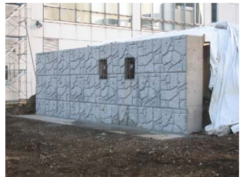
Photo 2 永久仕様の鉛直補強土壁 Permanent Retaining Wall
