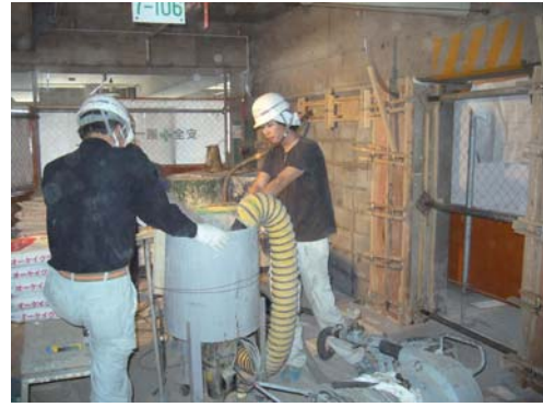
Photo 10 施工状況 Constructive Situation
