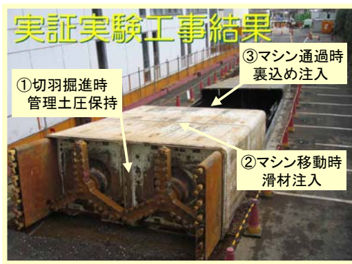
(a) 到達時のシールドマシン試験機の全景 1) Completion View of Shield Tunneling Excavation by URUP Matrix Shield Machine
