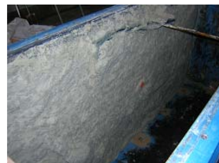
Photo 5 アクリル板背面の注入状況(ケース1) Situation of Inside Soil Tank After Injection Ends (Case1)
