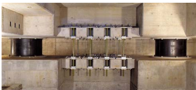
Photo 1 技研免震ビルの免震装置 Isolator and Damper Installed in the First Base Isolation Building of Obayashi
