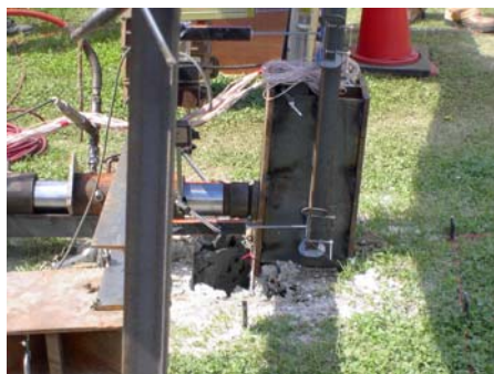
Photo 13 親杭の水平載荷実験 Horizontal Load Test of Solider Beam
