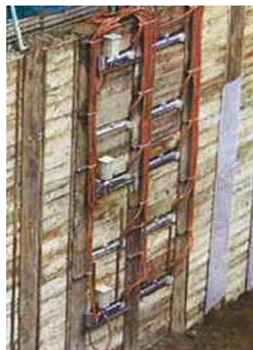
Photo 12 親杭横矢板の計測 Monitoring of Braced Wall with Solider Beam and Horizontal Board
