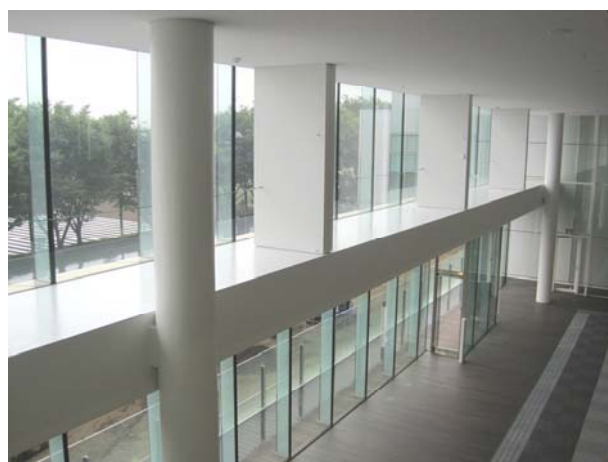
Photo 8 超高強度CFT柱の適用状況 Application of Ultra High Strength CFT Column
