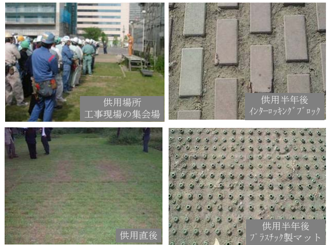
Fig. 2 従来技術の適用状況 Examples of Degradation of Past Greening Pavement
