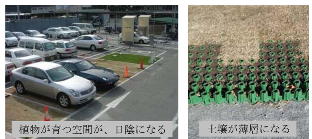
Fig. 2 従来技術の適用状況 Examples of Degradation of Past Greening Pavement
