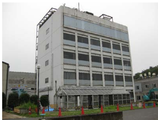
Photo 1 免震ビル Outline of Demolition Building
