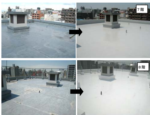
Photo 2 塗装前と塗装後の様子 Rooftop before and after Painting "Sun-Barrier"
