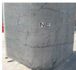
Photo 9 NE隅角部 Damage at the NE corner
