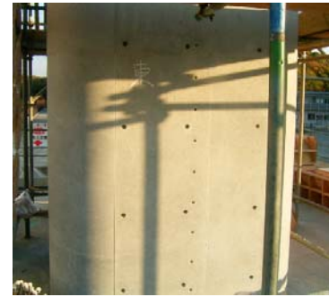
Photo 7 脚柱部の状況 (E-Defense) Column Mass Section
